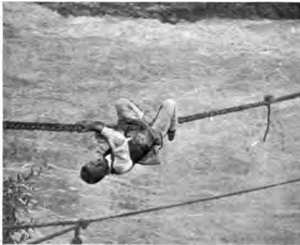
NATIVE CROSSING ROPE BRIDGE
